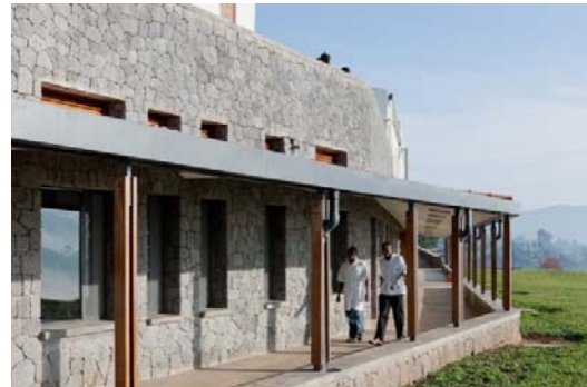
Figure 4: The hospital in Butaro, Rwanda (source: reference 9)
